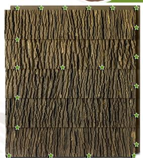
Step 9. Strike a chalk line to check that your course is level and begin installing the second course of bark shakes from the far left, beginning with a partial shake. Be careful to stagger seams between shakes so they do not line up with the course below.
